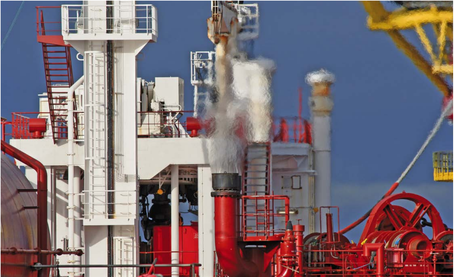
VOC release on a tanker loading from the Gullfaks field: GBA Marine's new system should reduce this substantially
