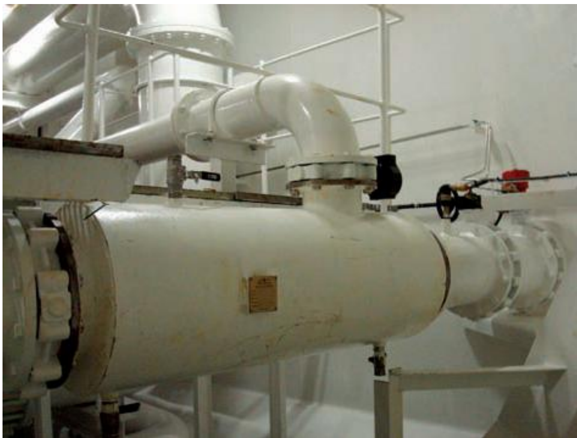
GBA Marine's Swirl Absorber seen fitted on board Navlon Hispania.
